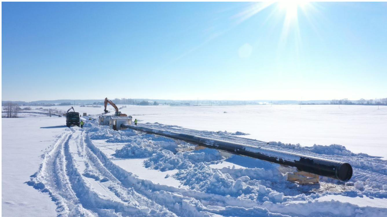
Works to connect the gas pipeline elements to the gas transmission information system are carried out at the starting point of the GIPL pipeline, next to Jauniūnai gas compressor station in Širvintos district. At the same time, the GIPL gas pipeline is being integrated into the control system of Jauniūnai gas compressor station.
